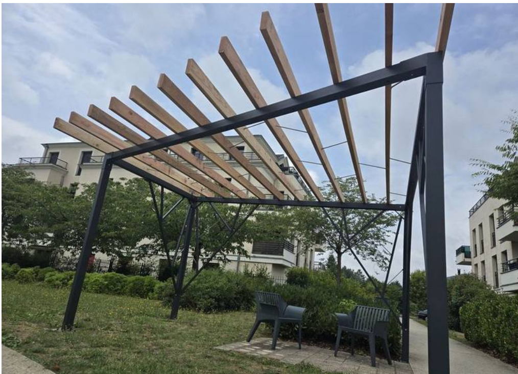
Pergola acier et lames bois, structure arborescente
